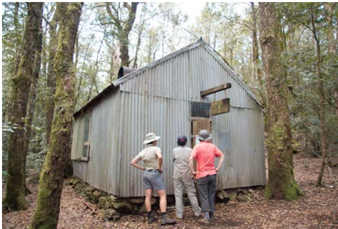
Inspecting the Selby Alley Hut
